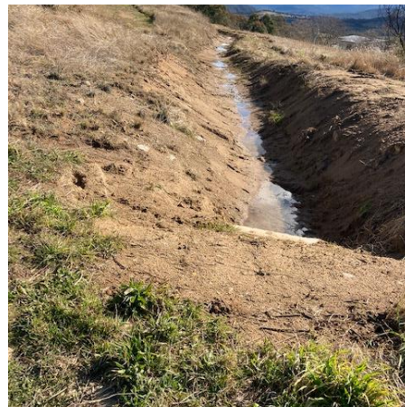
Cut drain maintenance Photo: Alan Ford
