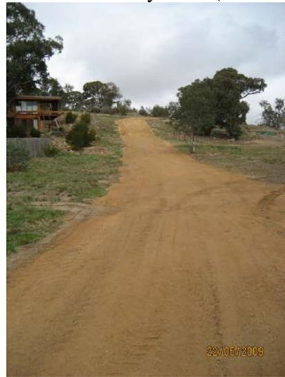
Paddy's River Granite was a convenient source of material for the job. Unfortunately, on steeper inclines, it was difficult to walk on without slipping. Much of the gravel eroded away (Photo 1) into the adjacent woodland.
