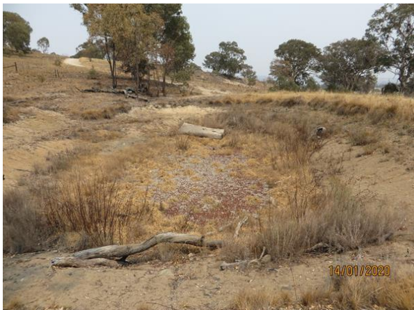
Kathner St Dam 14 January 2020 Photo: Malcolm Gill
