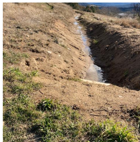
Cut drain maintenance Photo: Alan Ford
