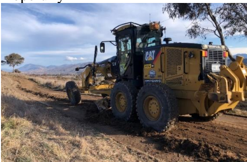
Grading the BNT Photo: Rob Lundie
