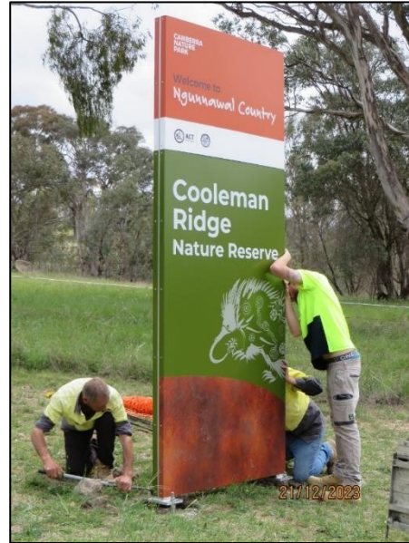
New sign being erected at Kathner St
